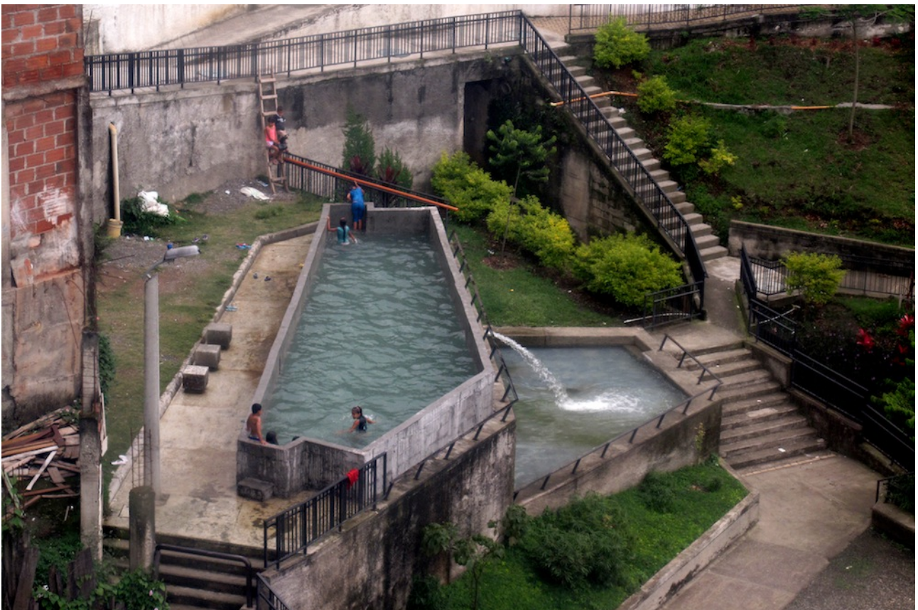
piscine a santo domingo
