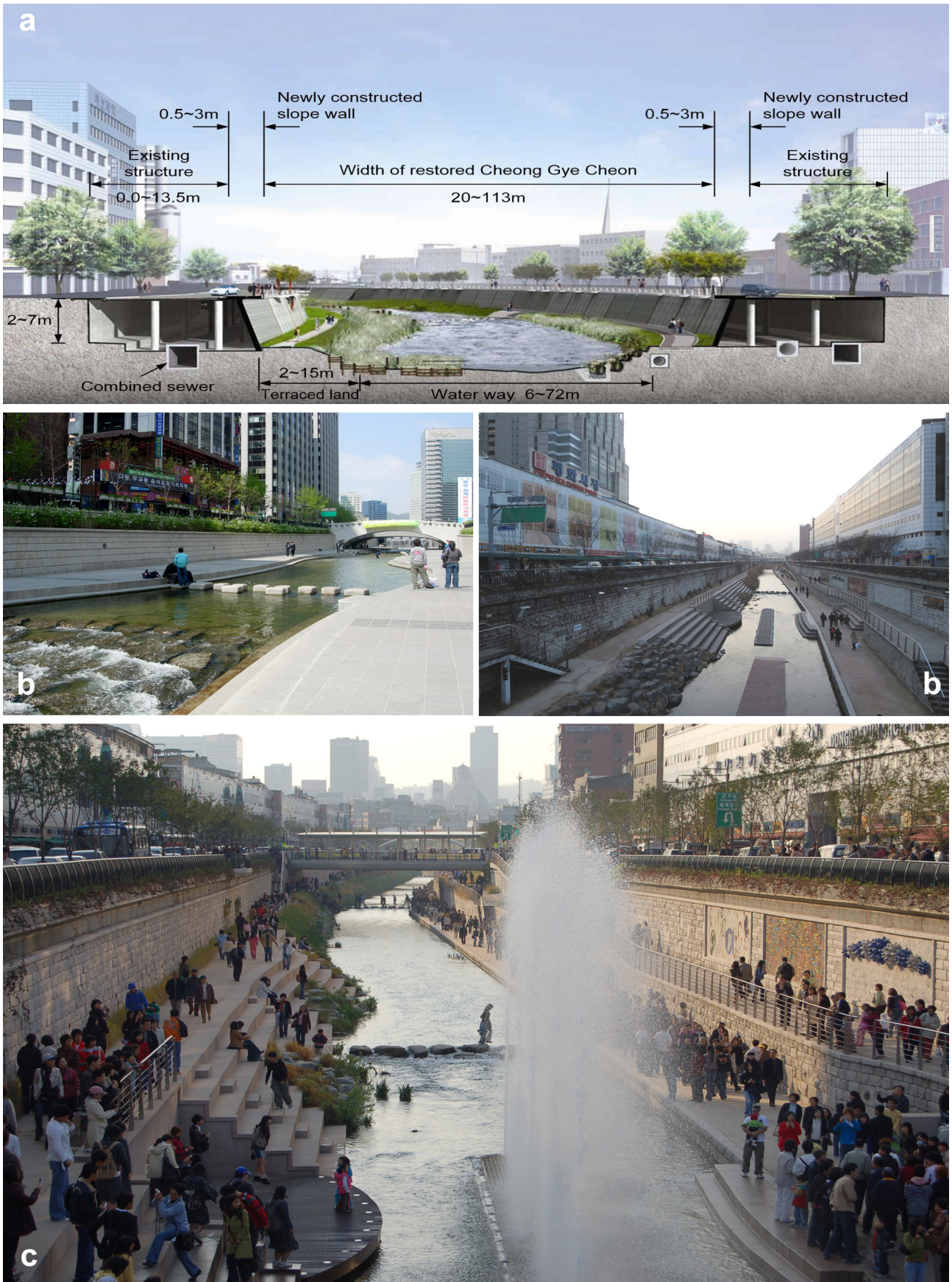
(Fig. 8) Cheong Gye Che , Seoul. Project by Cheongsuk Eng., Saman Eng. e Dongmyung Eng. + SeoAhn Total Landscape. 8a. Cross-section of the river restoration project; 8b; The restored riverbed between building and infrastructural pre-existences; 8c. A new co-evolutionary season for the story of Cheong Gye Che river.
