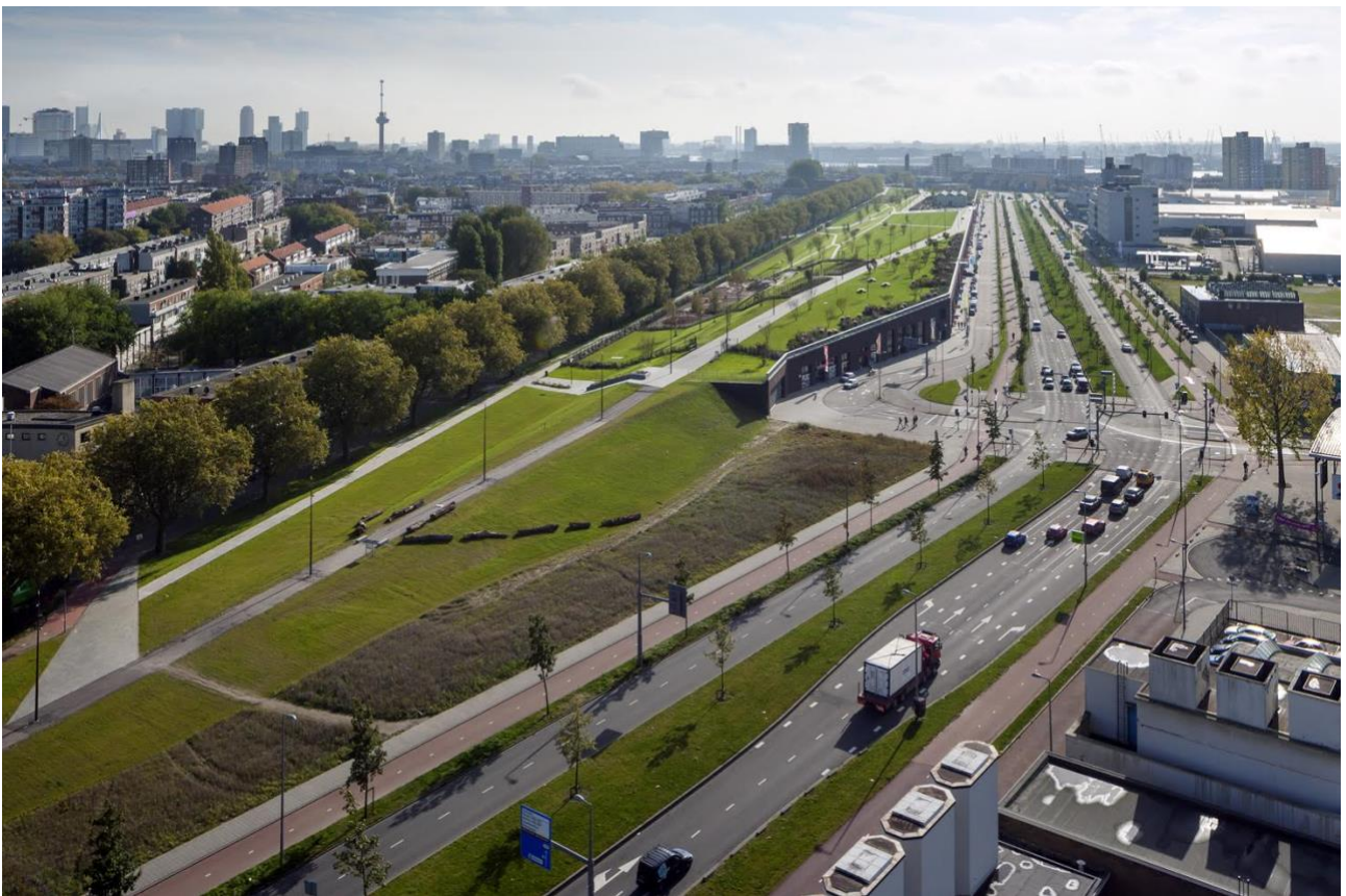
(Fig.1) The Dakpark from north-west in the 'harbour strip'. On the background: city center skyline. Author: Stijn Brakkee.
