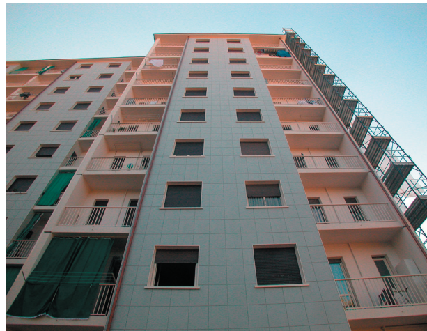
Fig. 3-3a. Strategies of refurbishment on the envelope. Use of ventilated façade in ceramic: the building before and after the intervention. (Credits: Silvia Brunoro)
