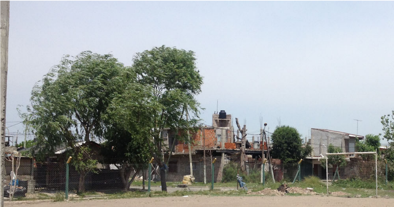
Fig. 4. Some buildings of the Villa along the riverside Reconstituta. In this area the risk of flooding is also connected to the issue of illegal dumping of waste from domestic ones, to those at high risk, such cars burned. The inhabitants of these places have a special relationship with the waste, since if they are from a hand a high source of pollution and disease, on the other hand are a resource to meet survival needs.
