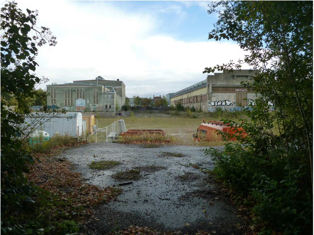
Jutier- und Tonnenhalle surrounded by urban wilderness (2011)
